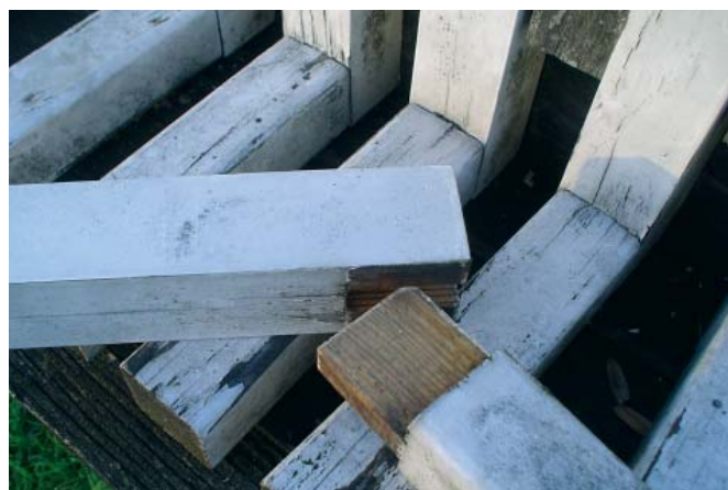
Figure 5: L-joints
